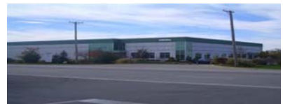
880 WOOD DALE, WOOD DALE • 48,242 SF +/- Divisible w/ 9,800 SF +/- Office • 6 Exterior Docks, 1 DID, 25' Clear Whse • Modern, Ideal Showroom/ Warehouse
