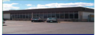
2100 BUSSE RD., ELK GROVE VILLAGE • 16,065 SF w/ 4 Mechanic Bays • 92 Auto and 70+ Trailer/Tractor stalls
