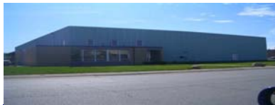
2195 ARTHUR AVE., ELK GROVE VILLAGE • 25,142 SF w/ 4,081 SF Office • 11 Exterior Docks, 3 DID, 18' Clear
