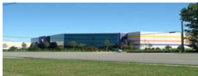
2315 LANDMEIER RD., ELK GROVE VILLAGE • 32,700 SF w/ 5,000 SF Office • 8 Ext. Docks, 1 DID, 25' Clear; Low Taxes
