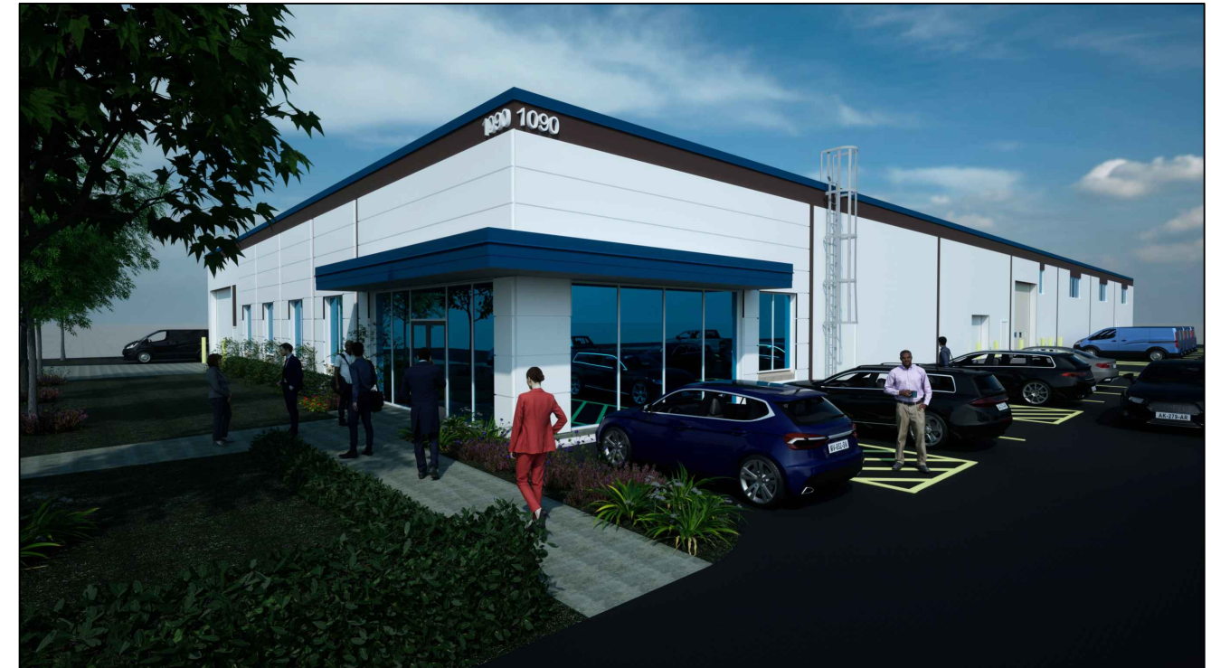
SOUTHEAST CORNER OF THE BUILDING
